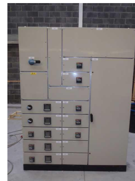
Figure 11 Form 4 Main Distribution Board
