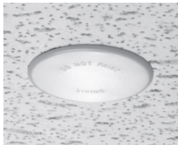
Figure 6 Residential sprinkler head
