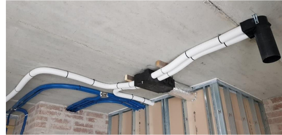
Figure 9 Apartment Ducting System
